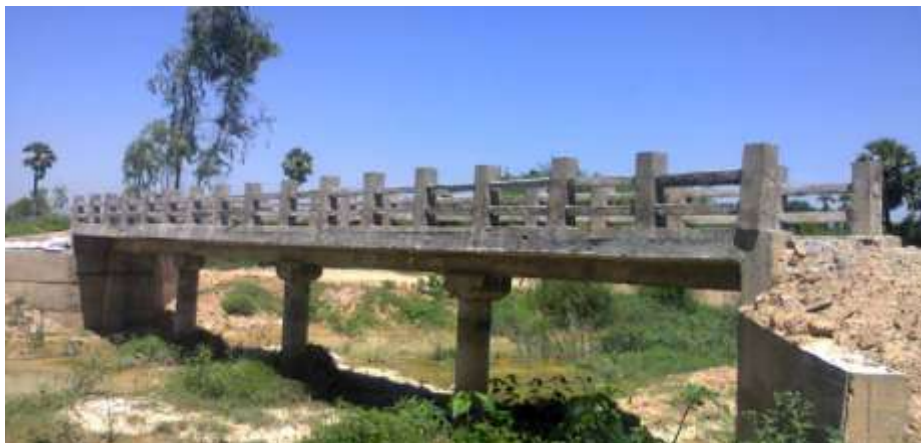
RCC Foot-Bridge Across Sengal Odai Stream Near Kalukanam Village
